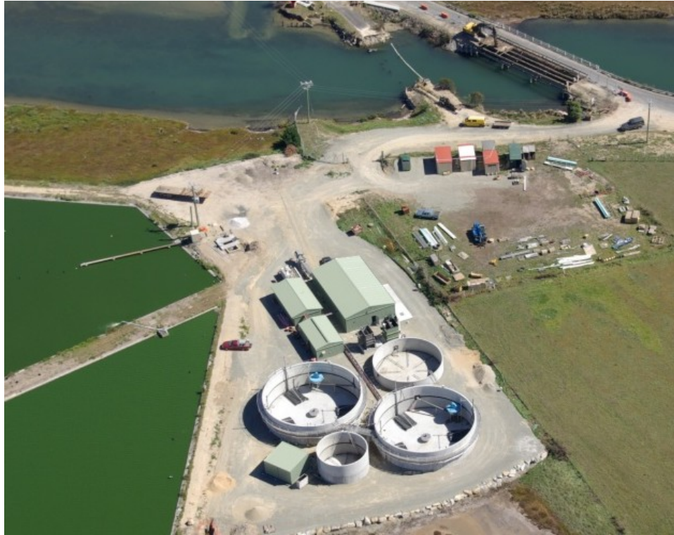
Figure 2. Aerial View of St. Helens MBTP
