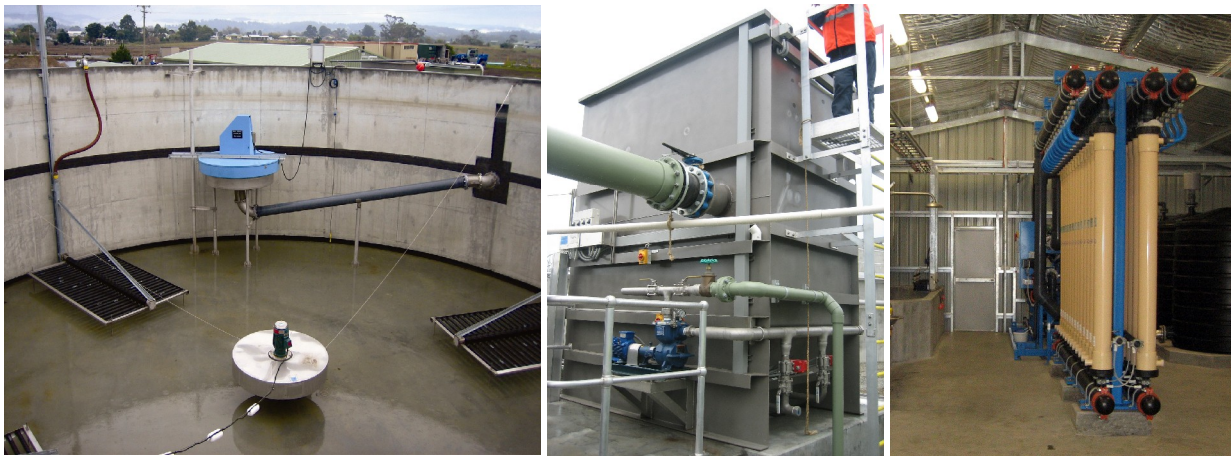
Figure 3. St. Helens MBTP – SBRs, CMF, and Membranes
