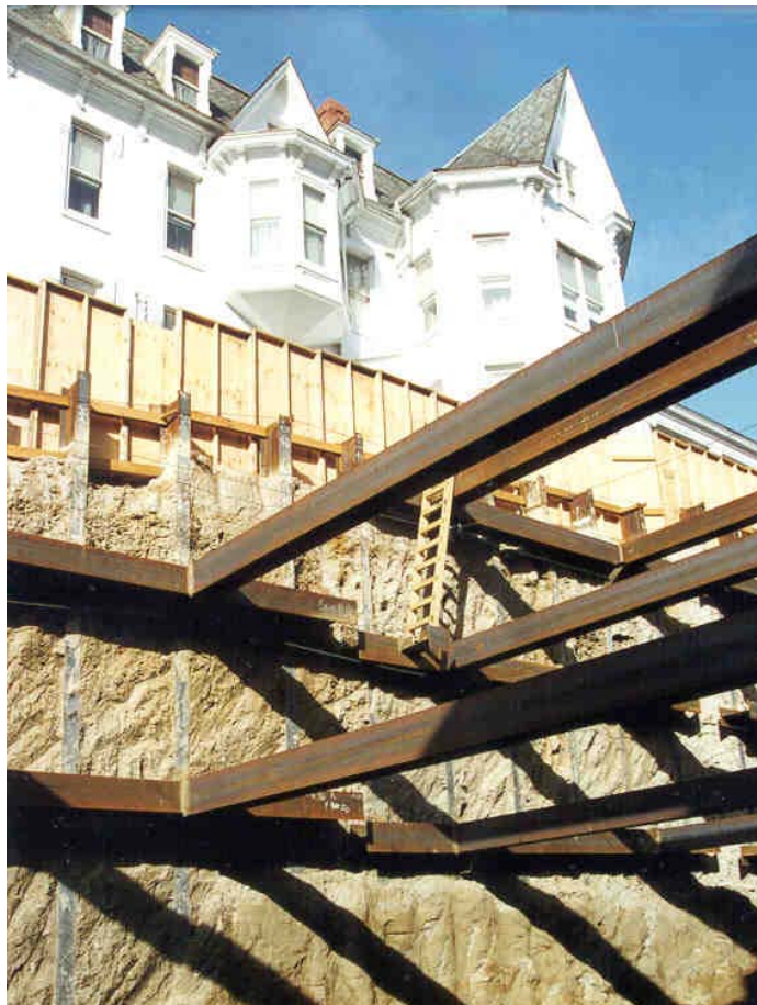
Figure 7. Deep Soil Mix Wall
